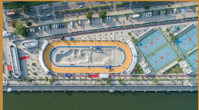
Sabarmati Riverfront Development Project
